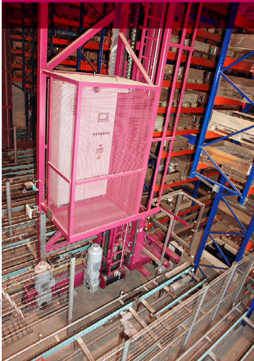
View into Liebherr's fully automated high-bay warehouse in Biberach
