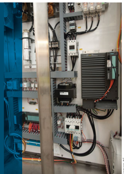
Simatic S7-300 and Sinamics G120 provide for the optimized control of water flow and pressure in the fountain
