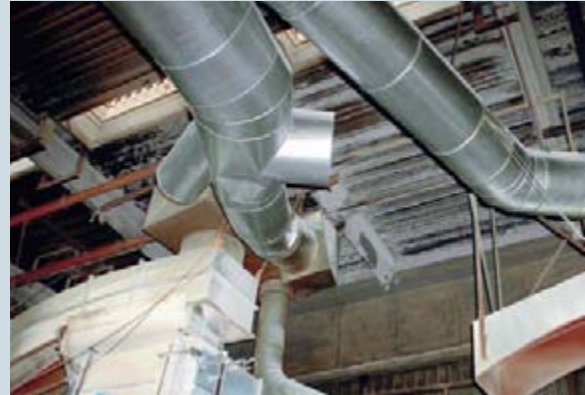
Inverters permit 66% energy savings in a flue-gas filter system at Siemens
