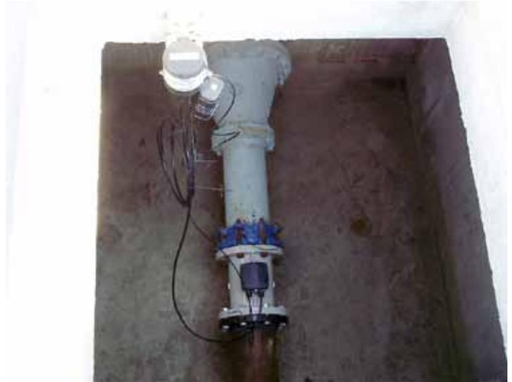
The Mag 8000 meter is a higher accuracy flowmeter that requires no maintenance and no power connection. It can be totally submerged with no effect on its operation.
