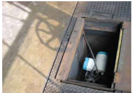
A coal-fuelled power plant in the United States automates the filling process of their coal bunkers by using a tripper car system and SITRANS LR460 to measure the level of coal in each bunker.
