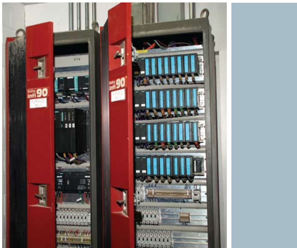
Cardinal Glass engineers say a big reason the Menomonie plant met its cold repair schedule was because they saved time by retrofitting the existing Bailey control cabinets with new PCS 7 hardware.
