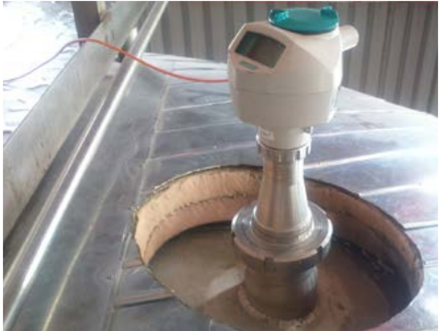
SITRANS LR250 measures accurately, even through foam conditions at SAB Miller.
