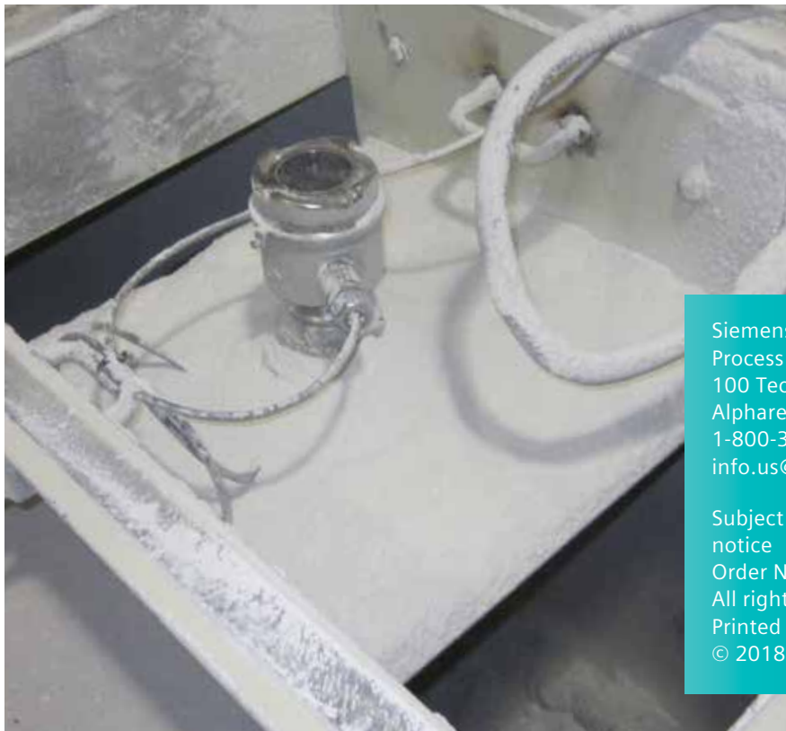
SITRANS LR560's highly durable polyetheramide lens antenna (left) can tolerate significant buildup, such as kiln dust
