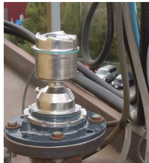
Figure 5: SITRANS LR560 avoids false echoes in a silo with its high frequency antenna, and no advance parameters are required for reliable operation.
