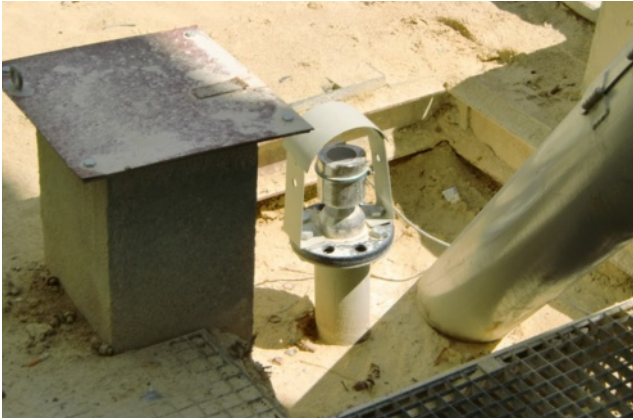
Fig. 1: SITRANS LR560 on the narrow limestone-meal silo. With its narrow 4° opening and 78 GHz frequency, the radar fill level transmitter is easy to operate
