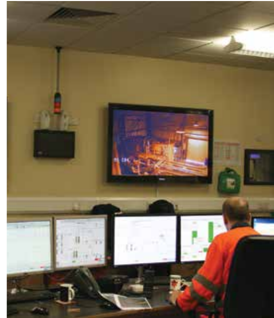
Using a SIMATIC WinCC SCADA System, operators monitor and control the entire facility from a central control room.
