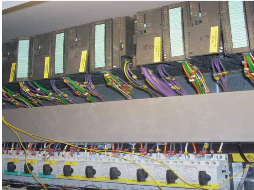
SIWAREX FTC weighing modules provide fast, continuous monitoring and control delivered directly to NOPA's control room.
