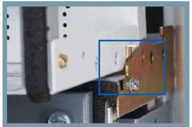
Up to three padlocks may be used to lock the disconnect handle in the OFF position. The unit is locked in the test position with one padlock. A copper clip on the side of the plug-in units engages the unit support bracket, grounding the unit at all times.
