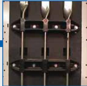
Standard isolated vertical bus design (rear view).
