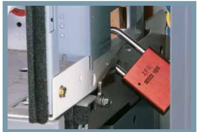
A screw driver operated defeater mechanism allows access to an energized unit by authorized personnel.
