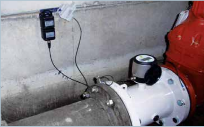
The MAG 8000 is flexible enough for installation virtually anywhere, including district water lines.
