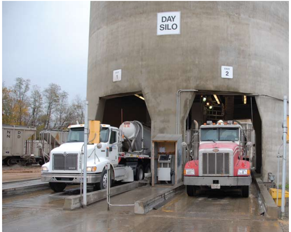
Day silo – Automatic truck loading operation
