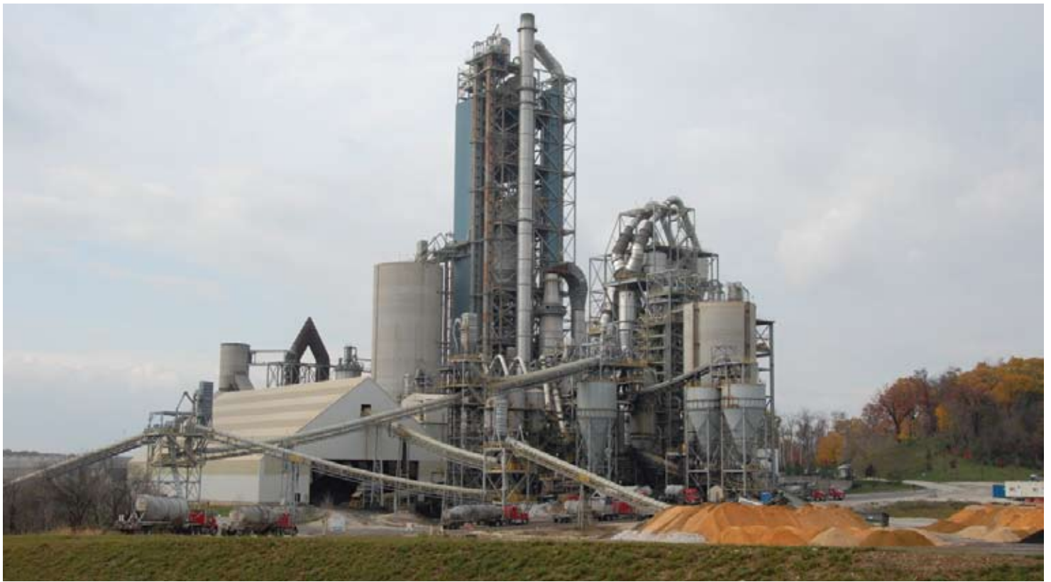
Lehigh Cement plant at Union Bridge
