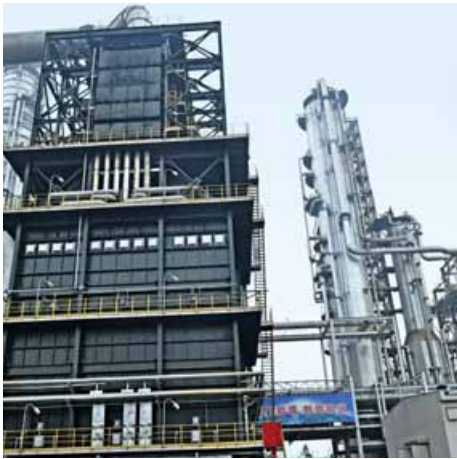
Siemens sets the standard for industrial control at the CNPC PetroChina mega refining and chemicals complex in Fushun
