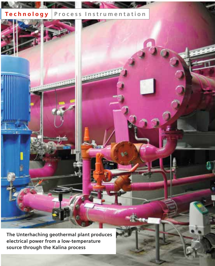
The Sitrans F C flowmeter monitors the ammonia-water ratio in the steam cycle
